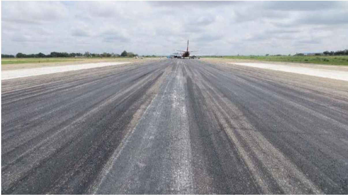
Figure 5: Rubberised deposits on the runway at DNYO
