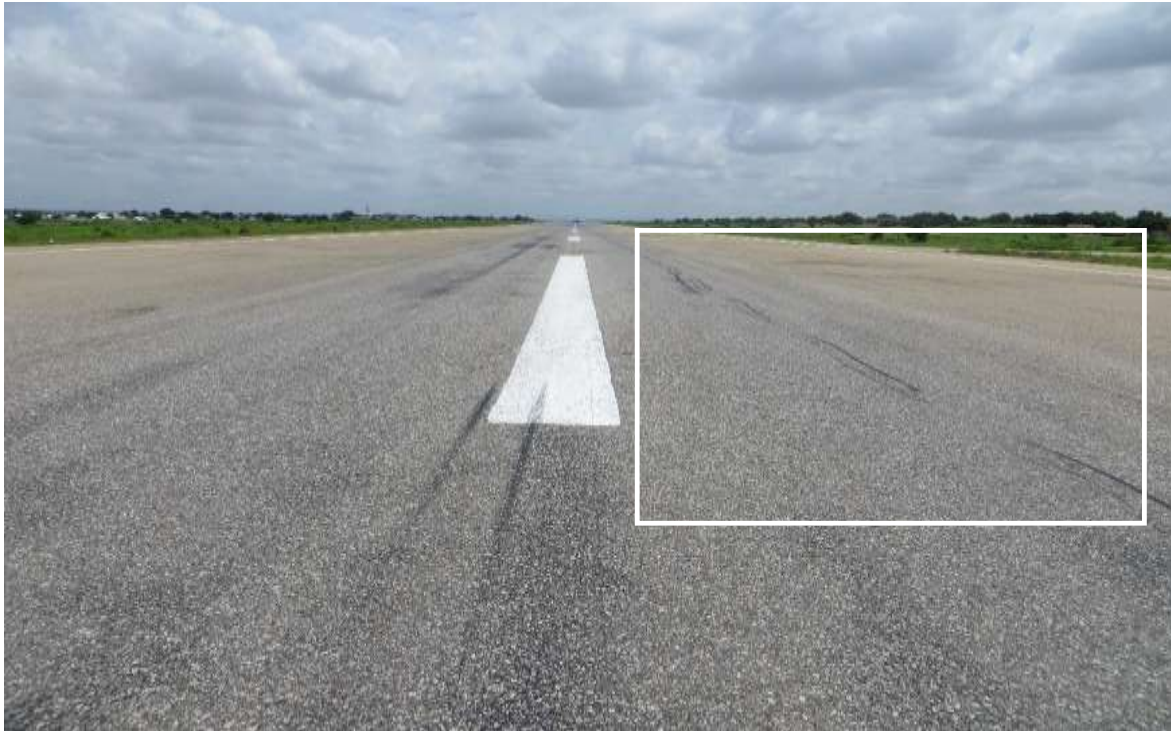
Figure 7: Witness marks indicating Tyre No. 3 failure
