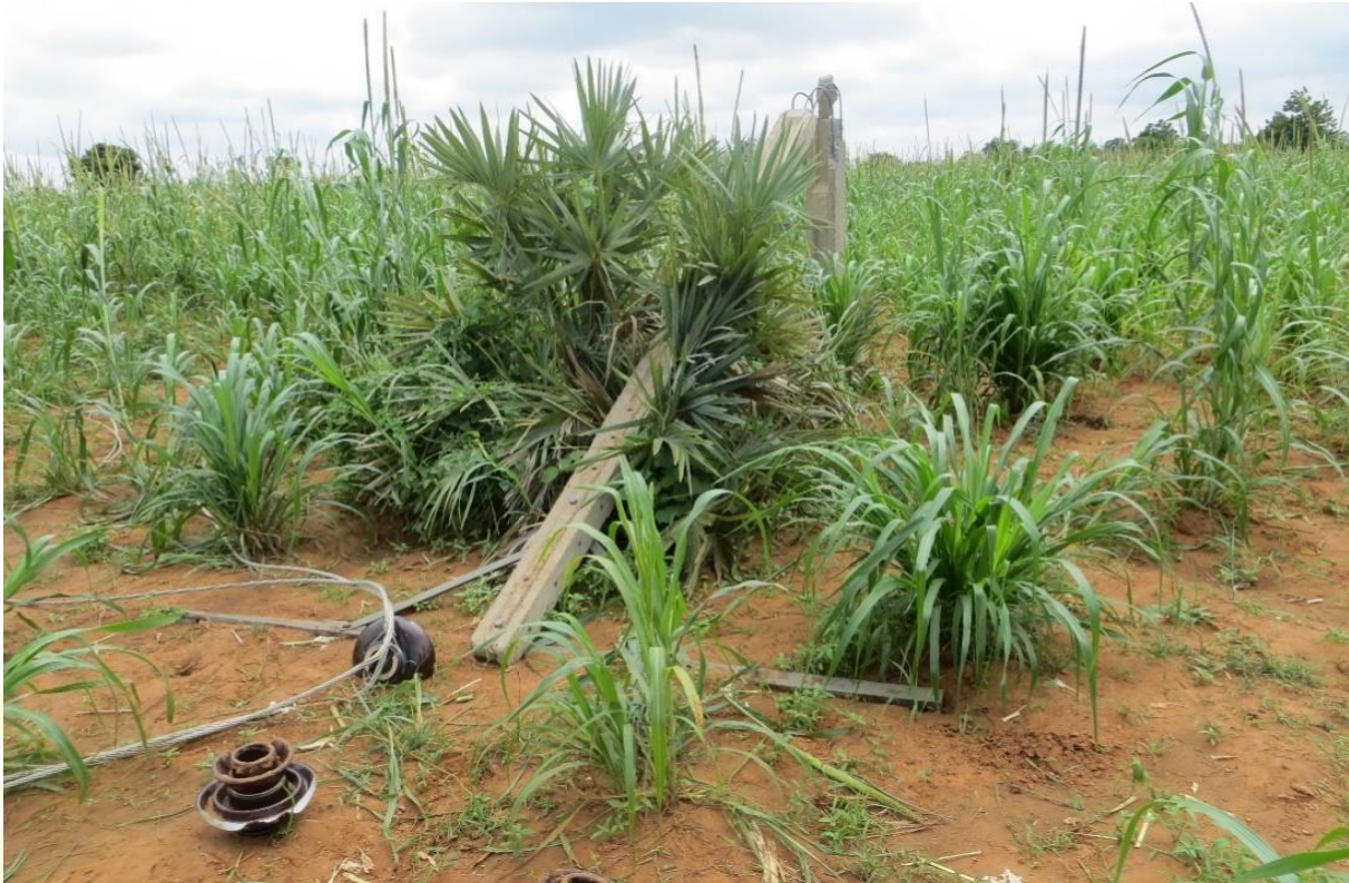
Figure 3: Electricity Distribution Concrete Pole brought down when the aircraft collided with the Power lines.
