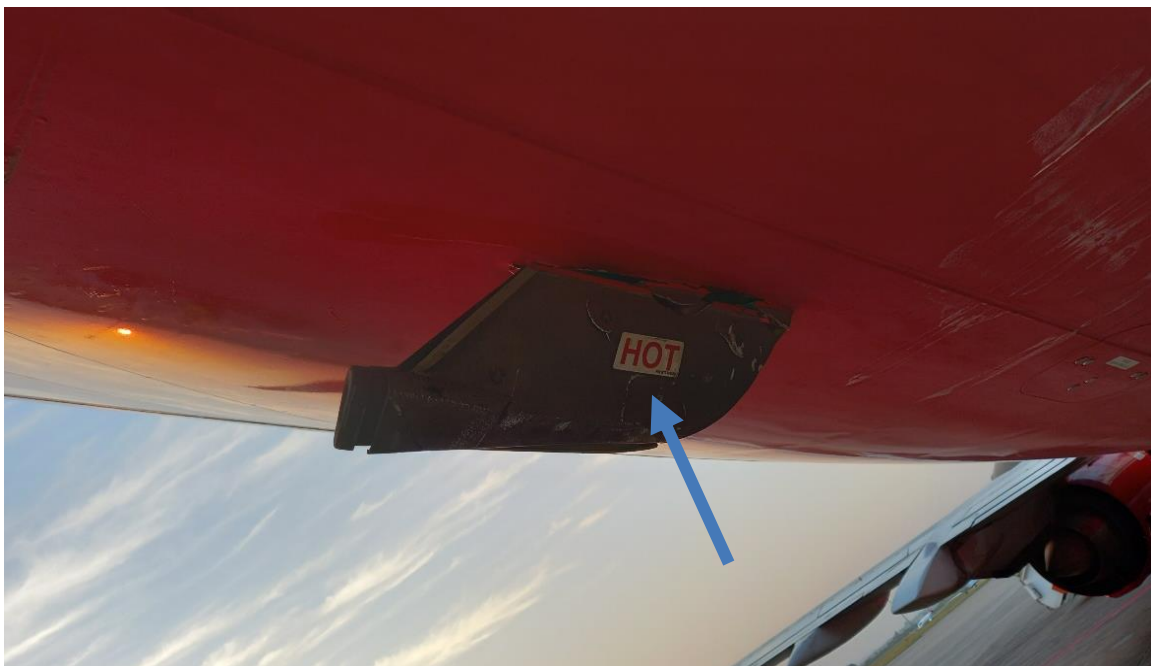
Figure 4: Damaged rear galley drains mast.
