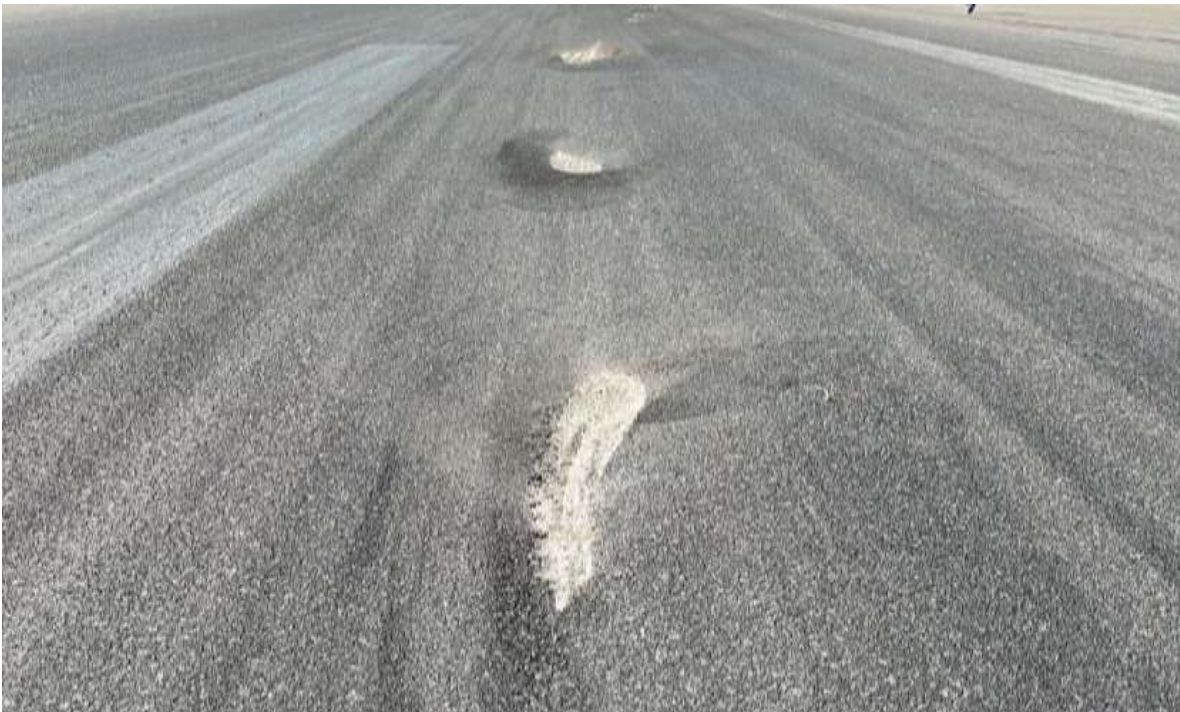
Figure 14: Multiple scratch marks on the runway surface
