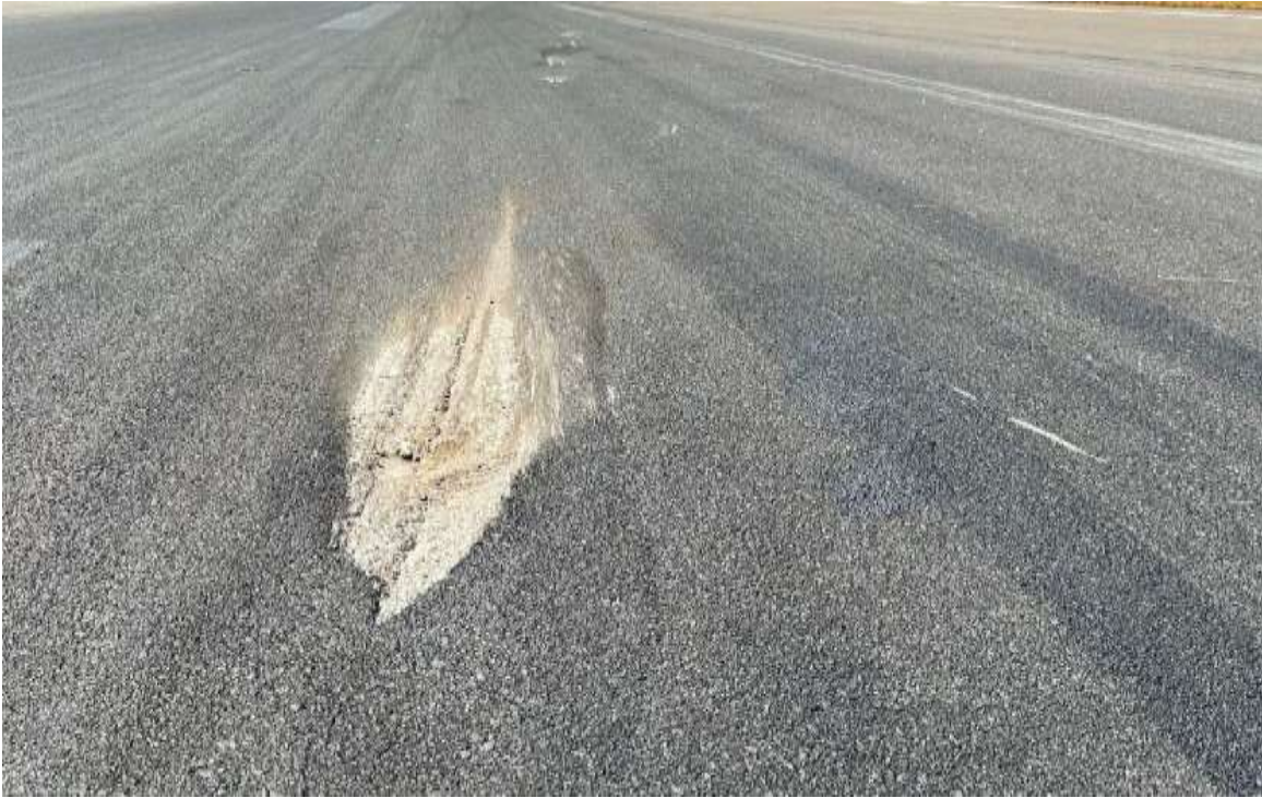
Figure 13: Scratch marks on runway surface
