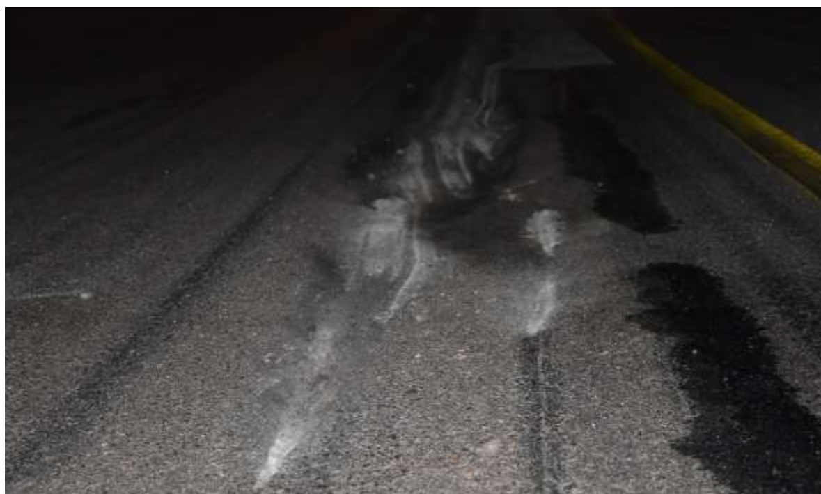
Figure 2: Scratch marks on the runway surface
