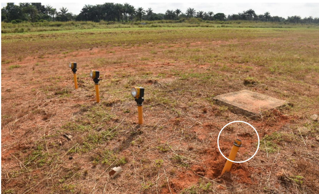
Figure 1: A damaged approach light on Row 11
