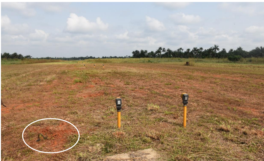
Figure 2: Another damaged approach light on Row 10
