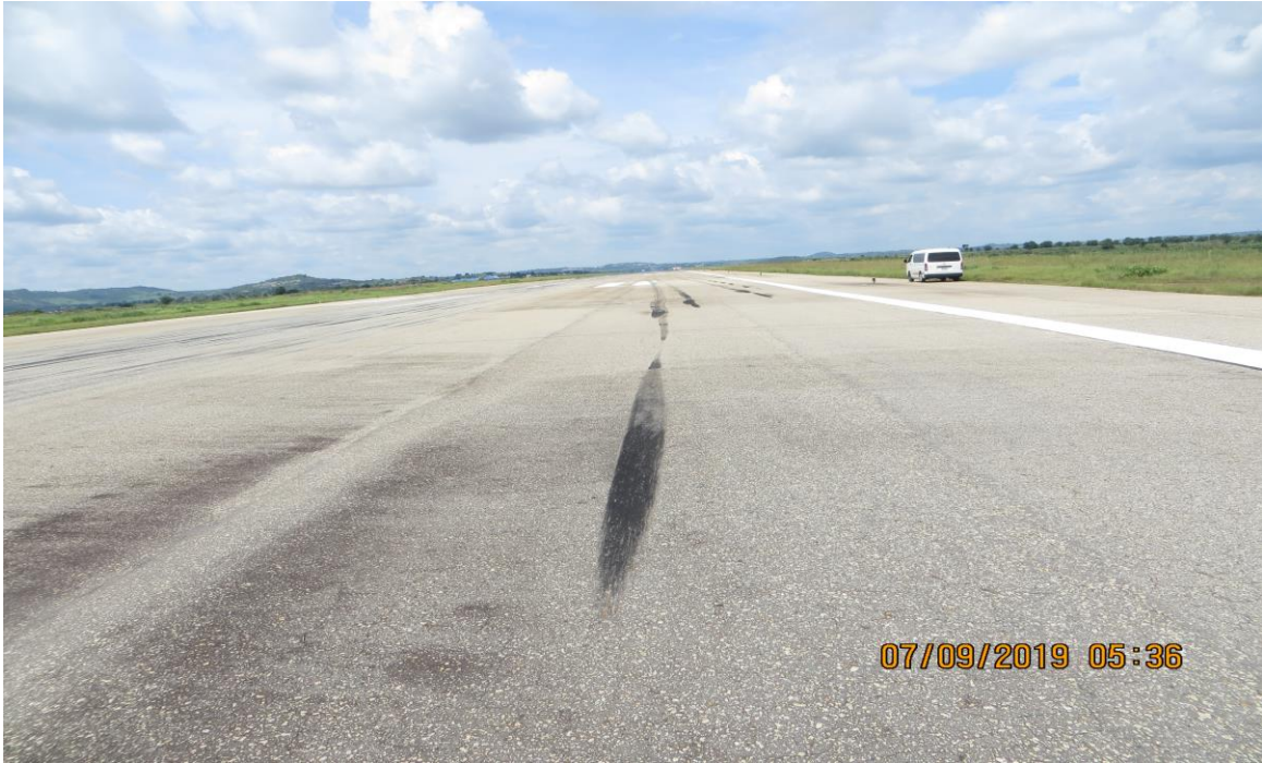
Figure 3: Tyre marks indicating the touchdown point
