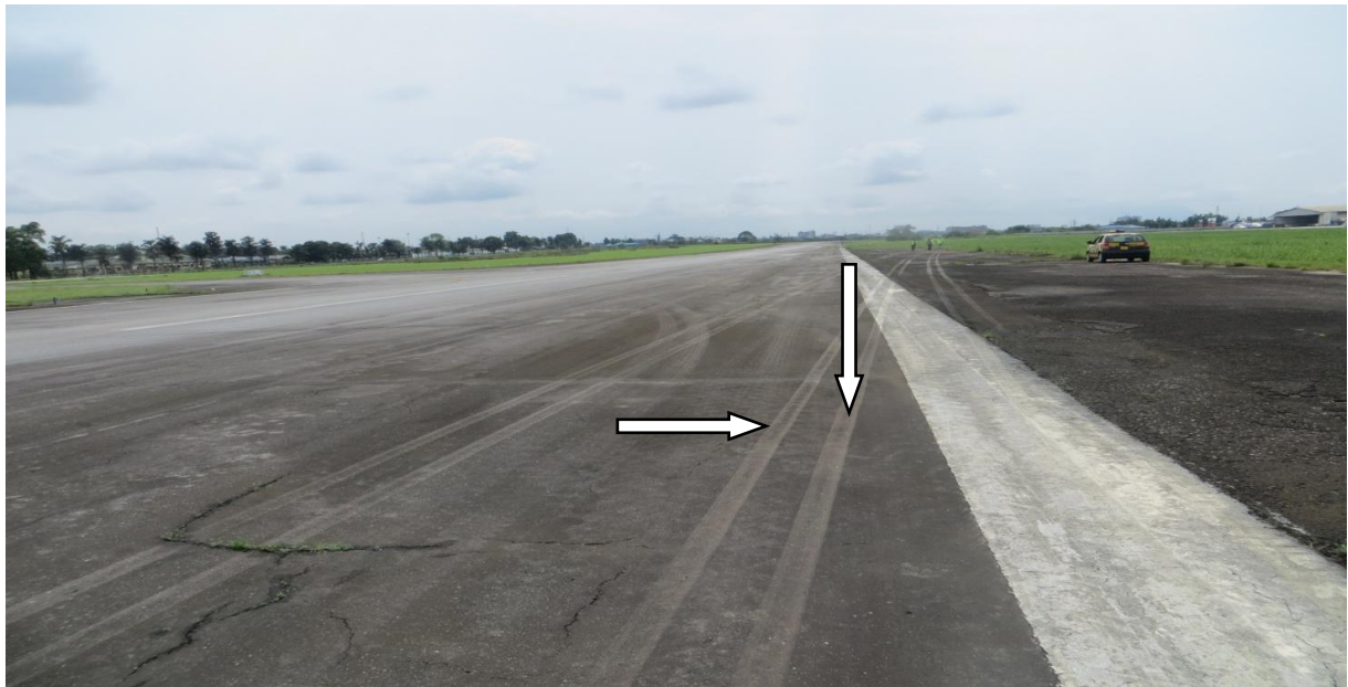
Figure 4: The aircraft main wheel tyre marks on the runway and the runway right shoulder
