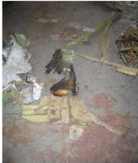
FIG 49 RBL 70.85 lower splice looking down and forward
