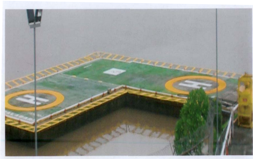
Figure 3: Addax Base Helipad, Calabar type, bearing strength in tons as 9.5 tons;
