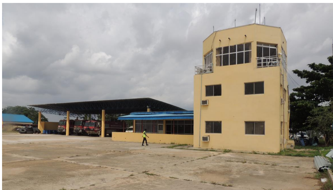
Figure 5: ARFFS Watch room/ATC Tower
