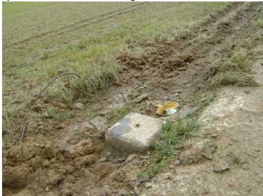
Fig 1.4 Damaged runway edge lights and uprooted armored cable
