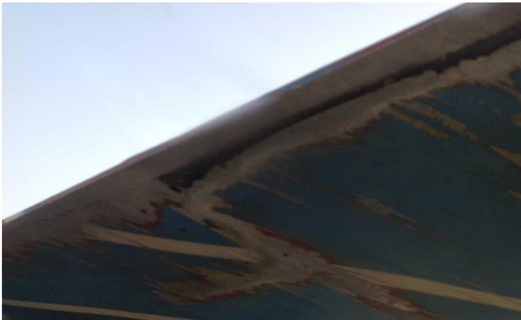
Figure 10: The torn right tank from the bottom
