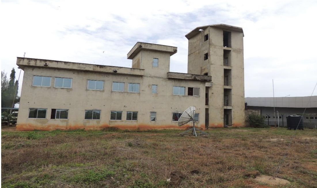
ATC tower under construction
