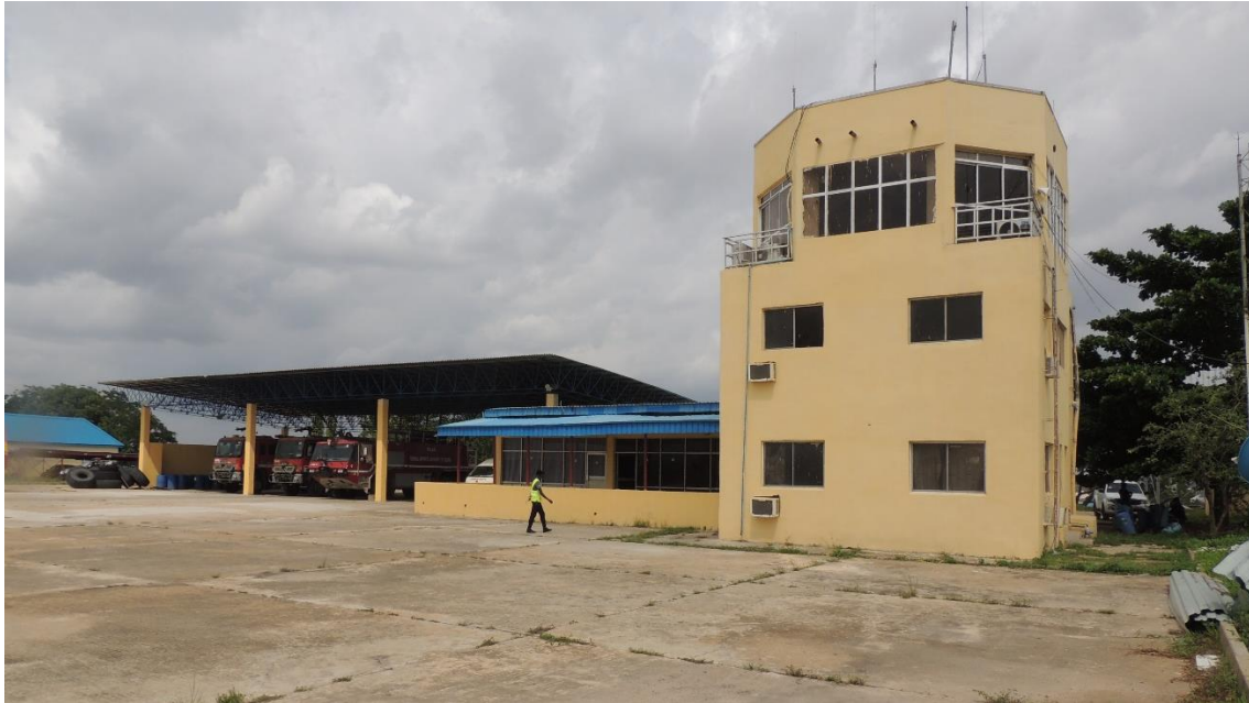
ARFFS Watch room/ATC Tower
