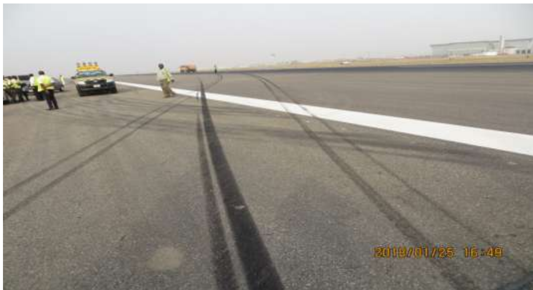
Figure 4: Picture showing tyre marks of the aircraft on the runway
