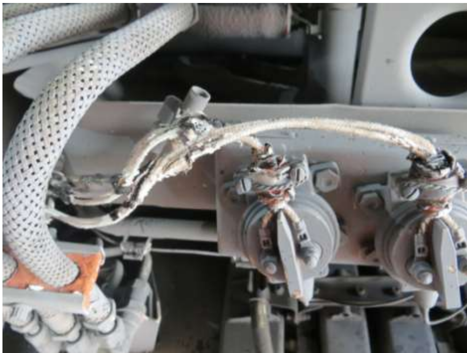
Figure 3: A close-up view of the charred wires
