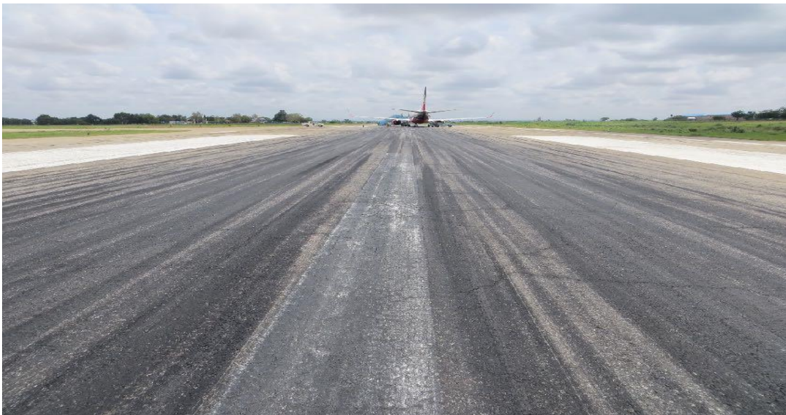
Figure 5: Rubberised deposits on the runway at DNYO
