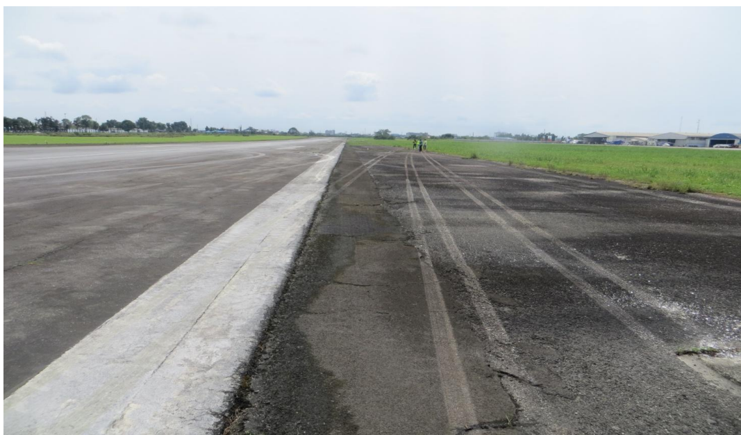
Figure 6: Photo showing the aircraft tyre marks on runway shoulder
