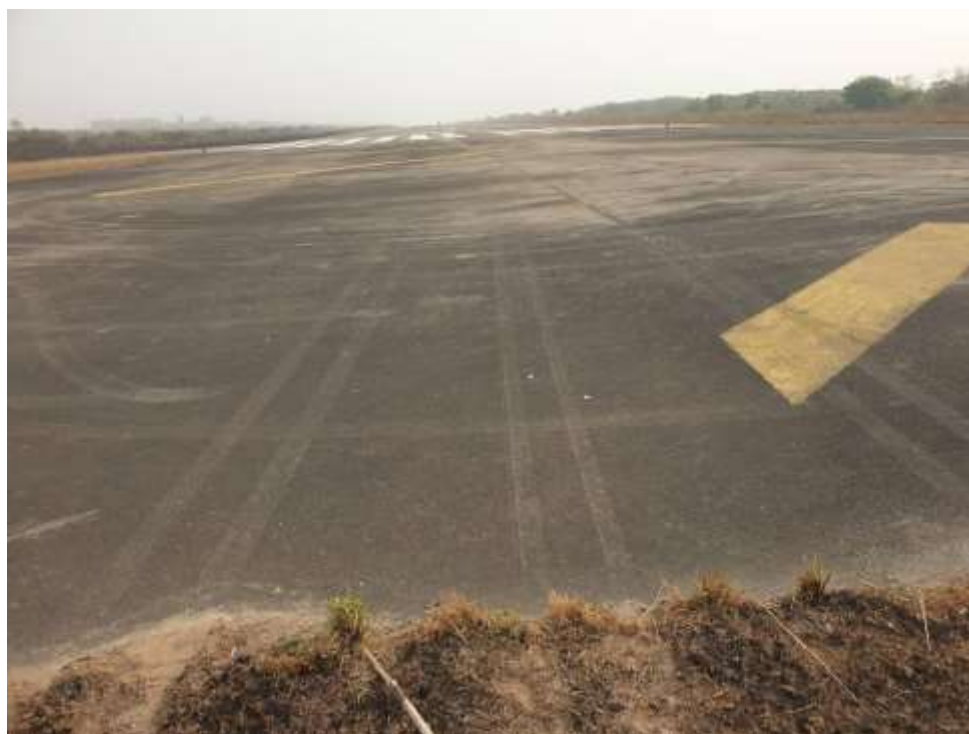
Figure 1: A view of the Runway 22 End Safety Area showing the aircraft tracks
