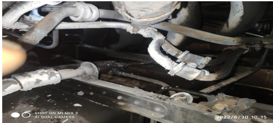
Photos showing severe fire damage to the left engine
