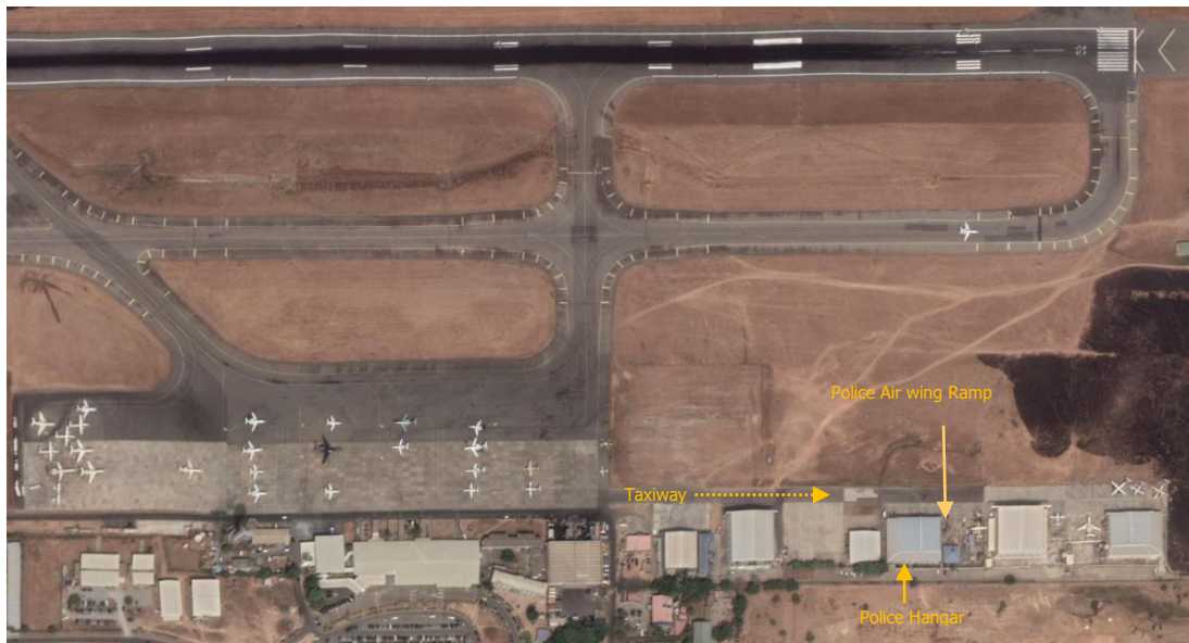
Figure 1: Aerial view of incident location. Source: Google maps.
