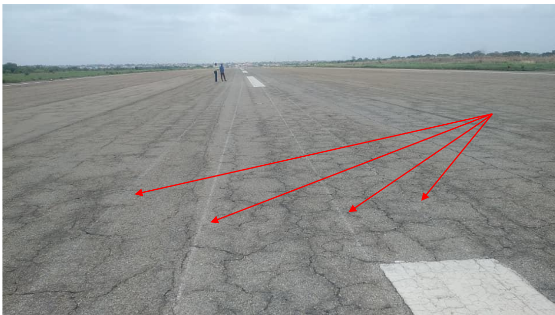
Figure 9: Photo of skid marks made by 5N-BNH on runway 23
