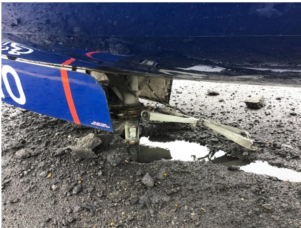
Figure 6: Photo showing nose landing gear strut with torsion link sheared off from lower end of the cylinder
