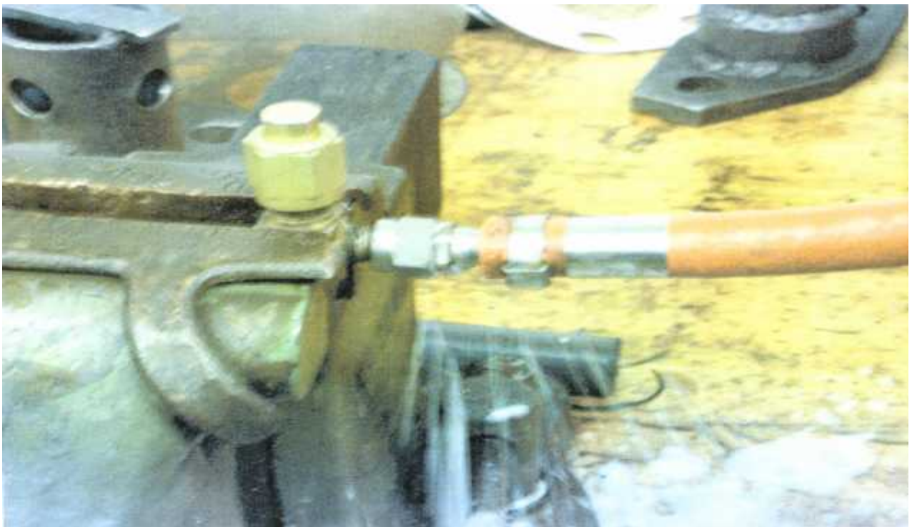
Fig.1-10 Photograph showing the hose leaking fuel under pressure
