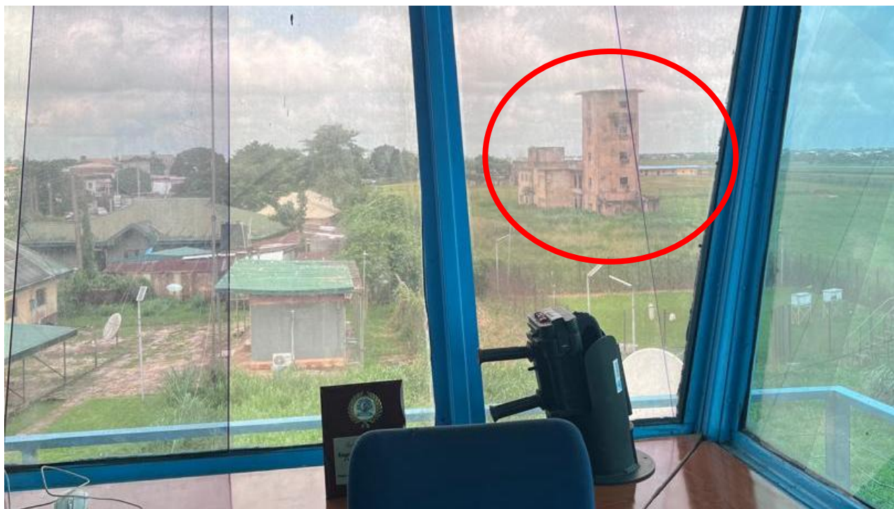
Figure 3: The incomplete building obstructing the line-of-sight to the end of Runway 05 (Runway 23 threshold end)
