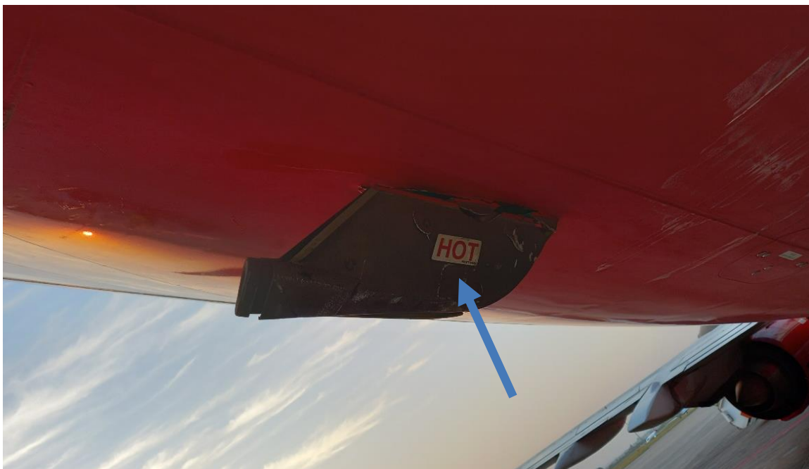
Figure 4: Damaged rear galley drains mast.
